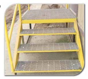
also provide easy passage of snow, light, air, water and moisture just as the original existing bar grating did for them in the past, while providing a slip resistant coating that allows for 100% shoe to surface contact.
