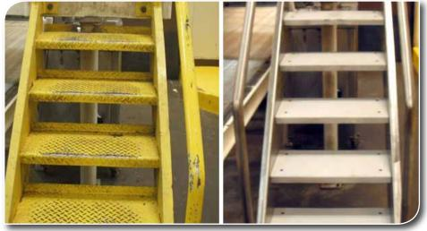
was a cost effective way to create an instantly safe surface that is lightweight and corrosion resistant without completely replacing the existing treads.
