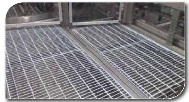
stair treads and grating were all galvanized after the slip resistant surface was applied. The galvanizing process allows for the steel surface to be protected against rust and corrosion.
