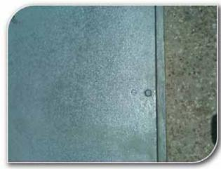
plate in place with flathead screws. *SlipNOT*<sup>®</sup> material can also be welded in place whether it is tack welding, seam welding or plug hole welding.
