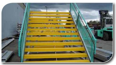
the slip resistant steps come into contact with oils, lubricants and coolants they will not corrode and will remain slip resistant. Furthermore, to create the safest work environment possible, Boeing painted the stair treads yellow. By painting the stair treads yellow, Boeing took preventative measures to ensure workers working on the stair treads would be noticed and that pilots moving planes would be aware of the location of the stair treads to prevent accidents.
