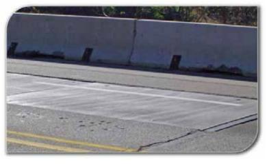
possible. *SlipNOT*<sup>®</sup> steel has a file hard surfce between 55 - 63 on the Rockwell "C" scale and has a bond strength of at least 4,000 psi, which provides a long lasting and durable surface. This became the most optimal choice for Ridgely Avenue Bridge because all *SlipNOT*<sup>®</sup> slip resistant products can be easily bolted and welded down to any bridge structure.
