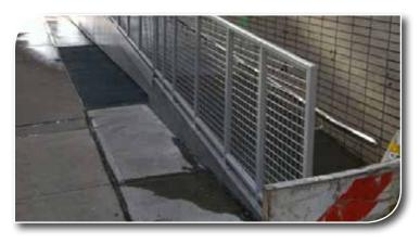
project, *Slip*NOT® provided 19 Pieces of various sized 1/2" Grade 3 galvanized steel plate, most in a 43 ¼" width; they were attached to the ramp with countersunk holes as specified in the drawings. Hot dipped galvanized plate was selected to provide corrosion resistance due to it being an exterior application with exposure to seasonal elements. The pieces were installed seamlessly to a stable platform and the access ramp had the appropriate flush transitions from the ramp to the platform.
